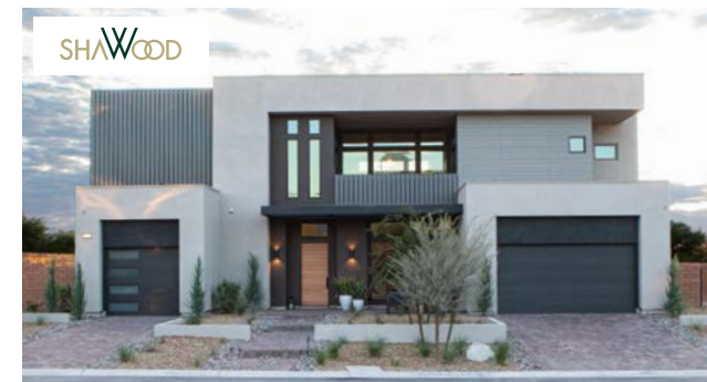
SHAWOOD pilot project in Las Vegas
